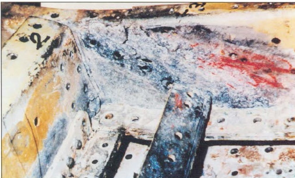
Figure 5-1. Corrosion Found After Removing Cargo Door Threshold Covers
